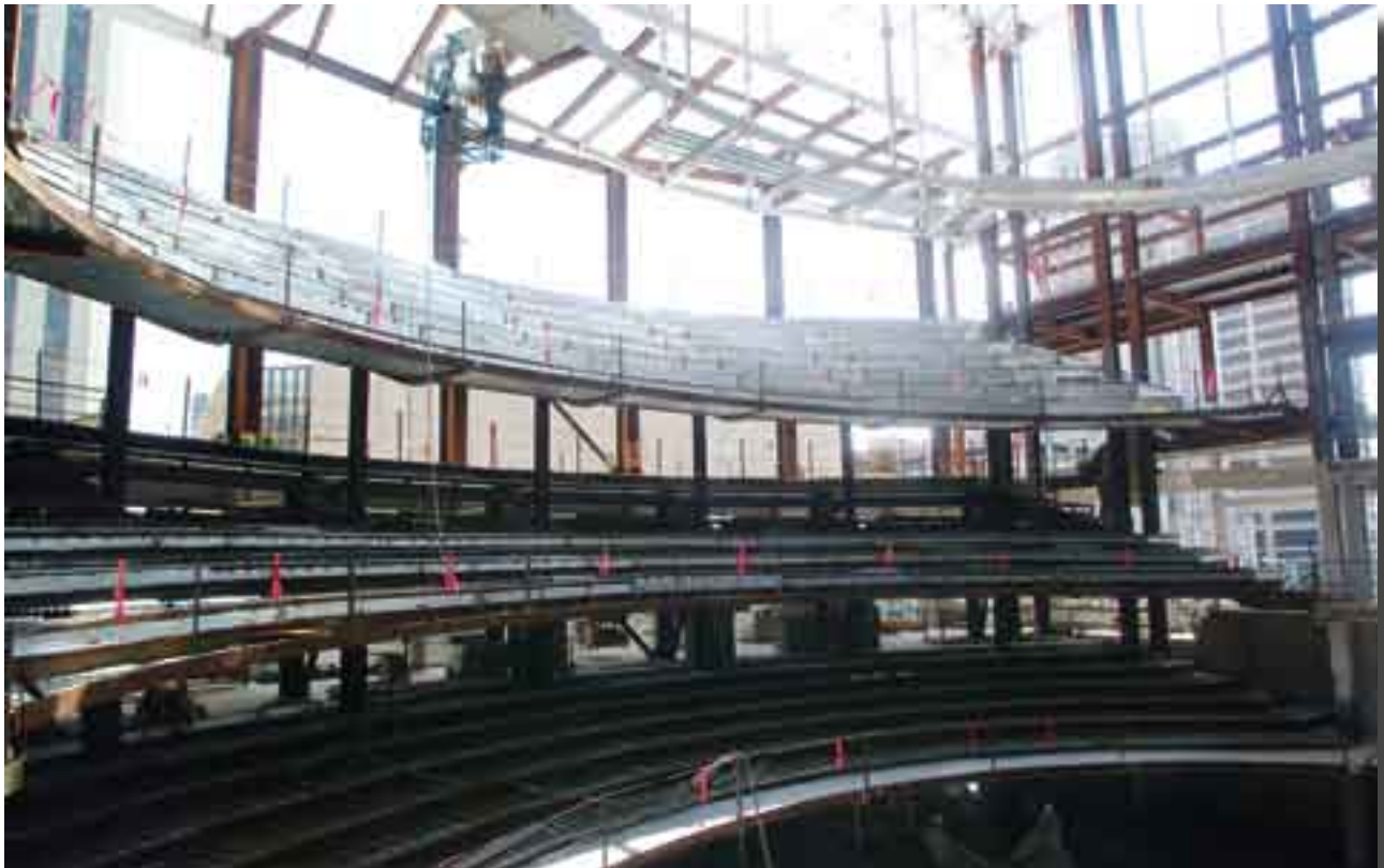
Construction of the balcony platform structures of Mead Theatre.
