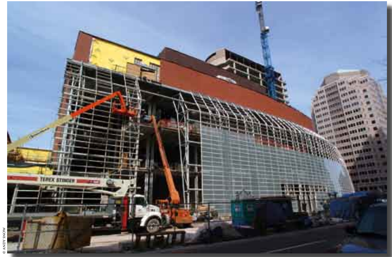
Wintergarden glass wall under construction during early fall of 2002.
